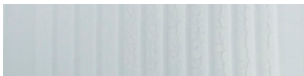
HEC Cracking > 14 Mils (0.36 mm)
